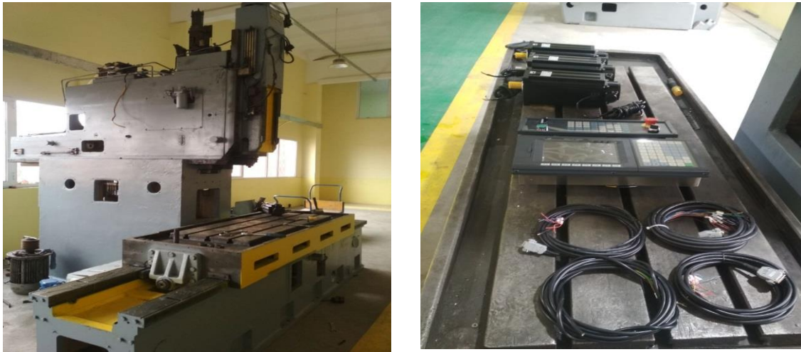
Fig 1.2. FP17SMN4 Vertical milling machine in the process of modernization.
